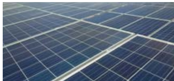
Modules at the centre of the site
