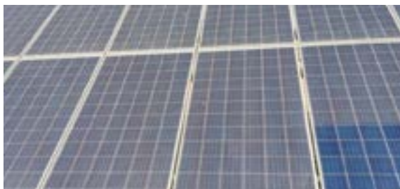
Modules at the boundary of the site
